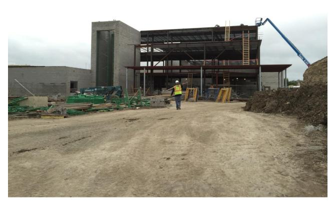
**LARGE GROUP INSTRUCTION (LGI)** – Steel roof decking is being prepared for roofing at the 3 story classroom building facing the north parking lot and Cedar St. The LGI classrooms are located on the first floor.
