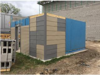
**QUALITY CONTROL MOCK UP BUILDING** – The wall water proofing, door and window flashing and exterior envelop materials are installed and inspected on a mock up prior to installation on the new building. The mock up is reviewed by the architect and SISD's 3<sup>rd</sup> party inspector. Once approved the mock up becomes the standard for installation on the building.
